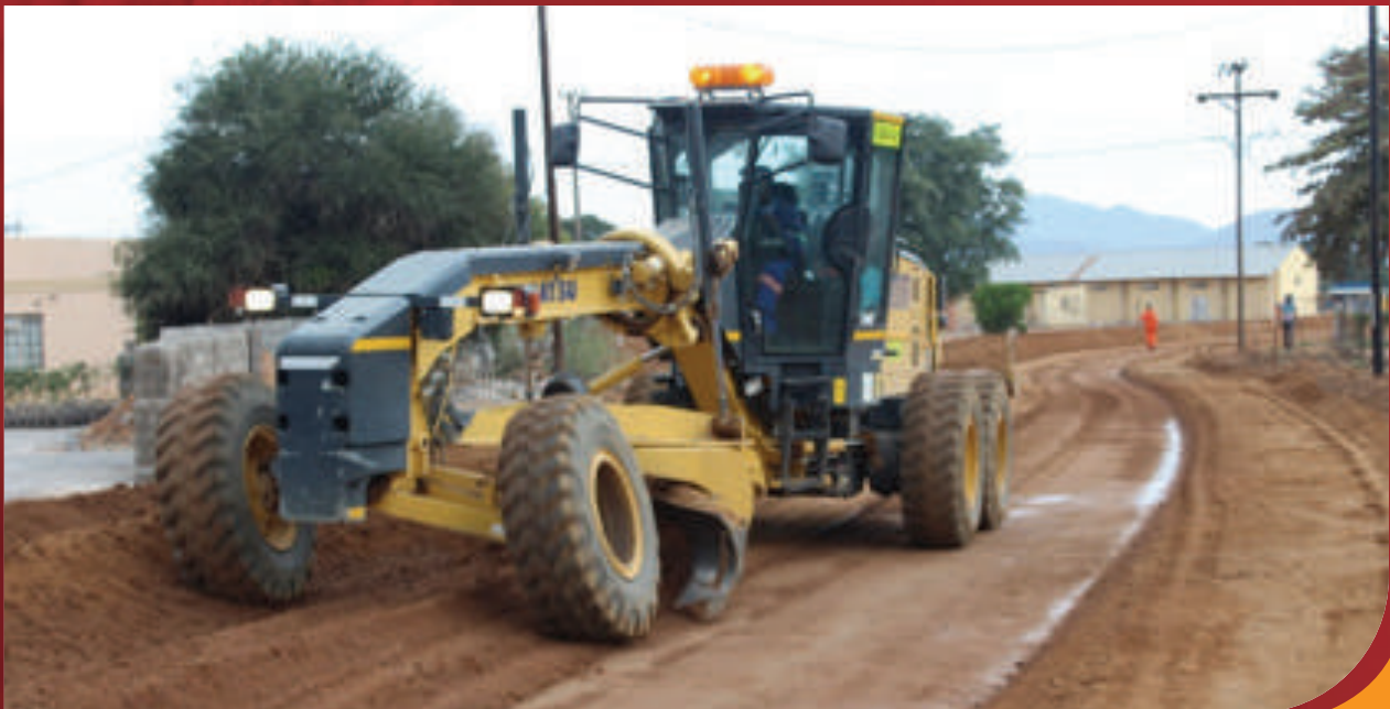
An Infrastructure Project In Botswana
